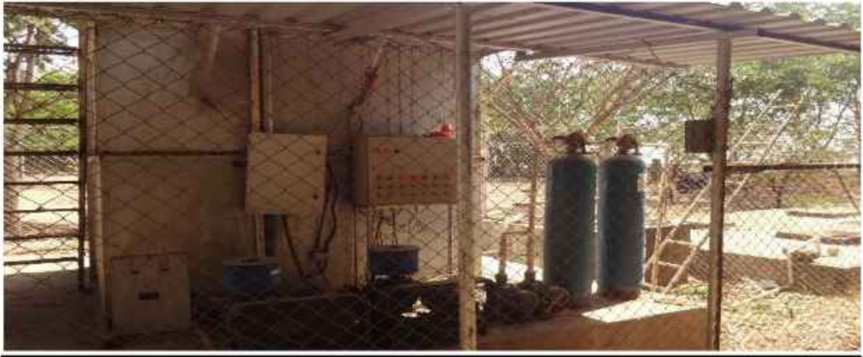
Assembly of Sewage Treatment Plant
