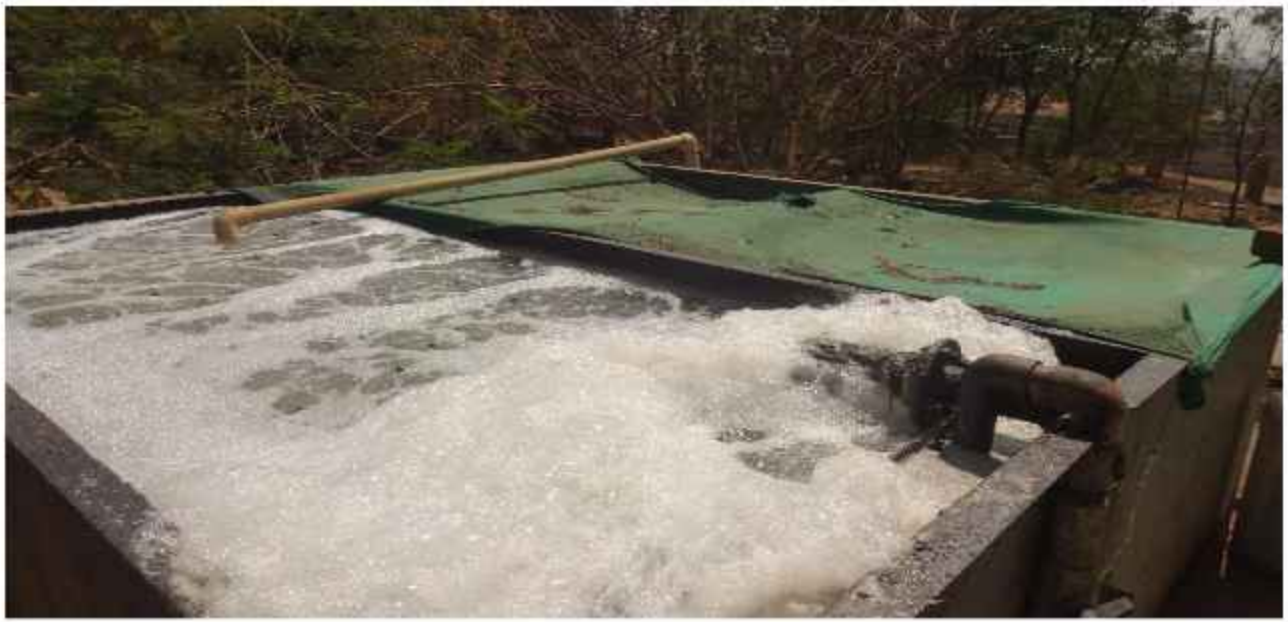
Sewage Treatment Plant
